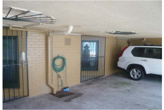
Figure 3.12 The Hughes Lane garage undercroft at 122-124 Victoria Street, Potts Point.
