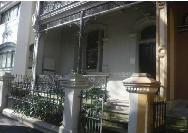
Figure 3.13 The historic front entrance to 120 Victoria Street, Potts Point.
