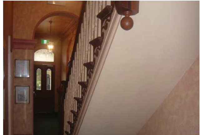
Figure 3.24 The timber staircase and front hallway at 122 Victoria Street, Potts Point.
