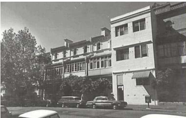
Figure 2.8 Photograph depicting the subject buildings in 1975, showing that the balconies of all three buildings had been enclosed by that date.
