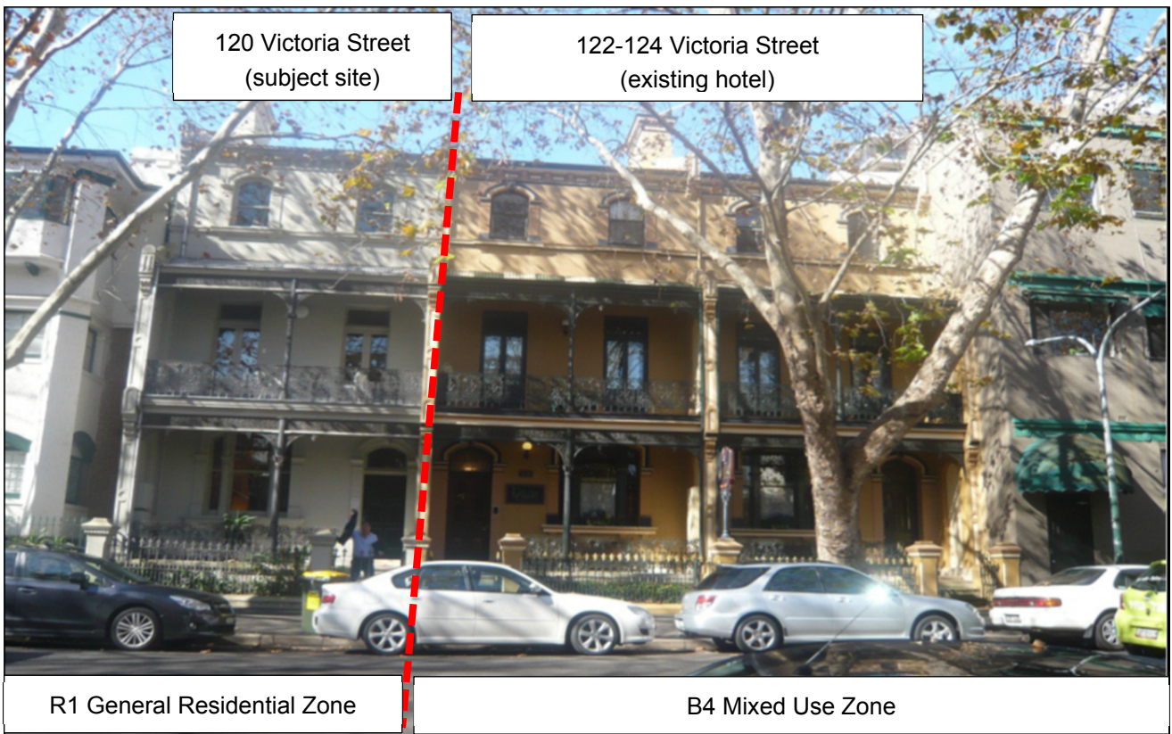
Figure 7: 120 to 124 Victoria Street, Potts Point with zone boundary shown dashed in red
