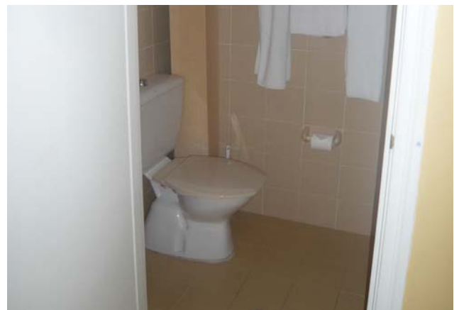
Figure 3.26 Modest bathrooms have been inserted within each existing guest room at 122-124 Victoria Street. This intervention has had the effect of altering the rooms' original symmetry and layout.
