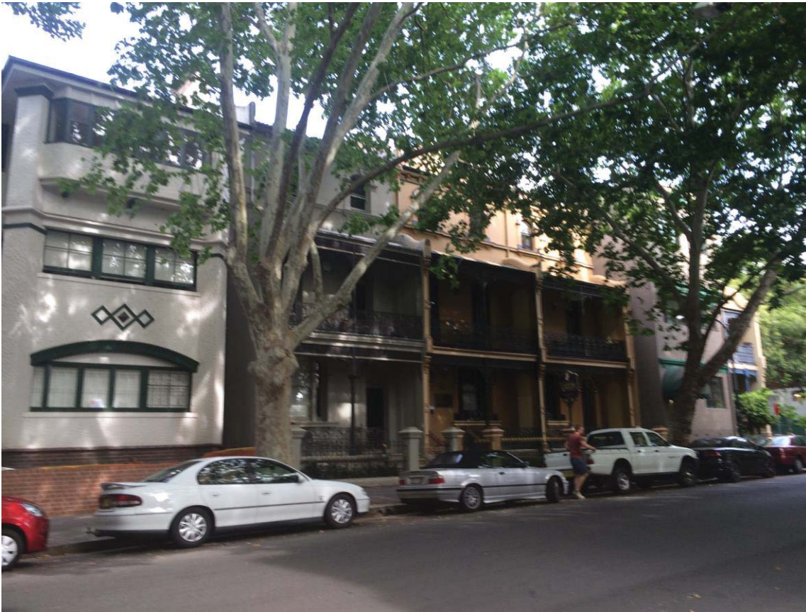
Figure 3. The subject site and adjoining Victoria Court Hotel (122-124 Victoria Street)
