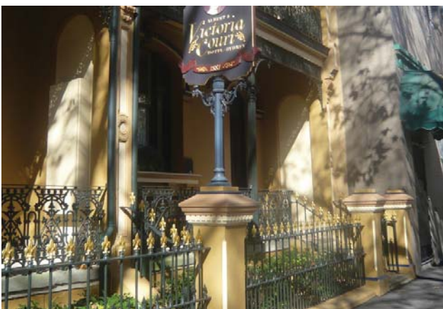
Figure 3.15 The historic front entrance to 124 Victoria Street, Potts Point.
